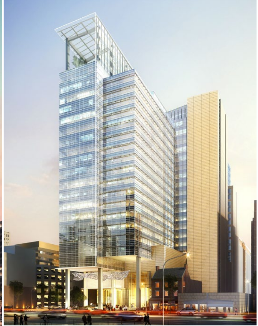
VIEW FROM WISCONSIN AVENUE
